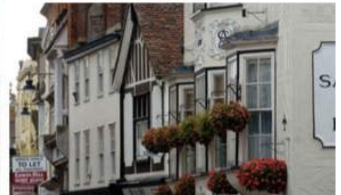
Historic street frontage details
